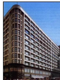
19. Almacenes Carson. Sullivan, 1889.
