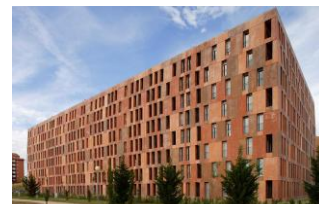
8. Viviendas Villaverde, Madrid (D. Chipperfield, 2005).
